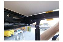
Rotate the yellow clips off one at at time starting from the bottom. Place the clip over the vinyl with the opening facing the ground and gently push downward so the clip starts to naturally rotate, continue in a rotating motion until the clip "clicks" into place. Repeat for all eight clips.
